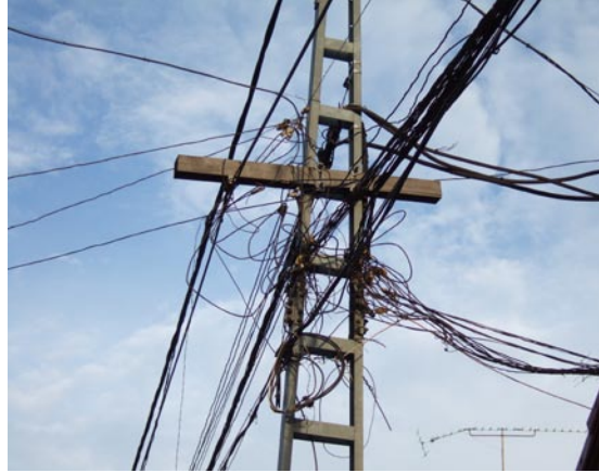
Fig. 169 and 170 Many developing cities, such as Vientiane (Laos), have limited street infrastructure. A street conversion can be the ideal time to make upgrades.
